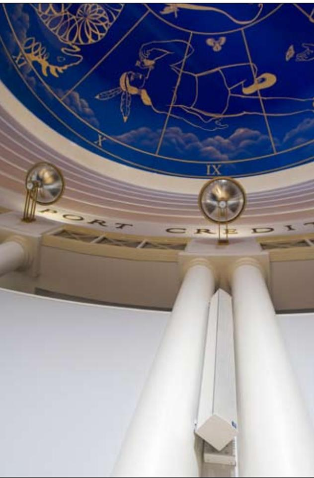
steer the sound directly to the audience without any splashing into the ceiling." An additional benefit is that the beams significantly reduce feedback from open mics directly in front of them.
