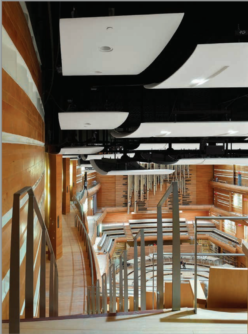
The reflectors seen above serve to distribute sound energy down to the stage and throughout the audience.
